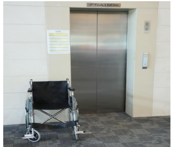
Lifts and wheel chair facilities
